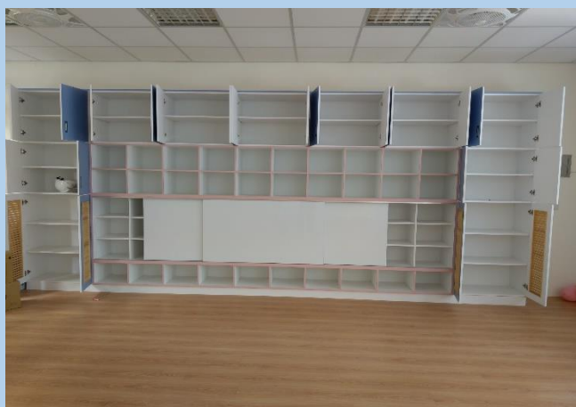
輕隔間擡擺(含掛勾及置物板)
