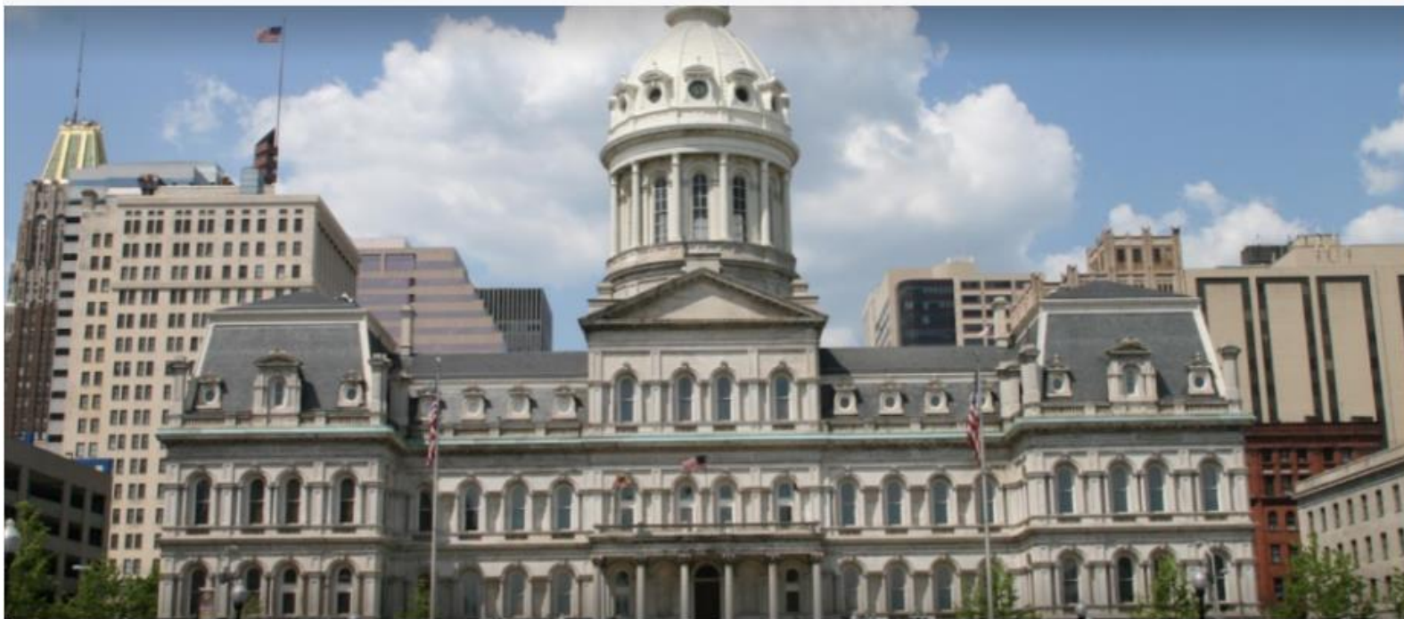
Baltimore City Hall · Photo by Ashley Hughes on Google maps ( shorturl.at/iMNV0 )
